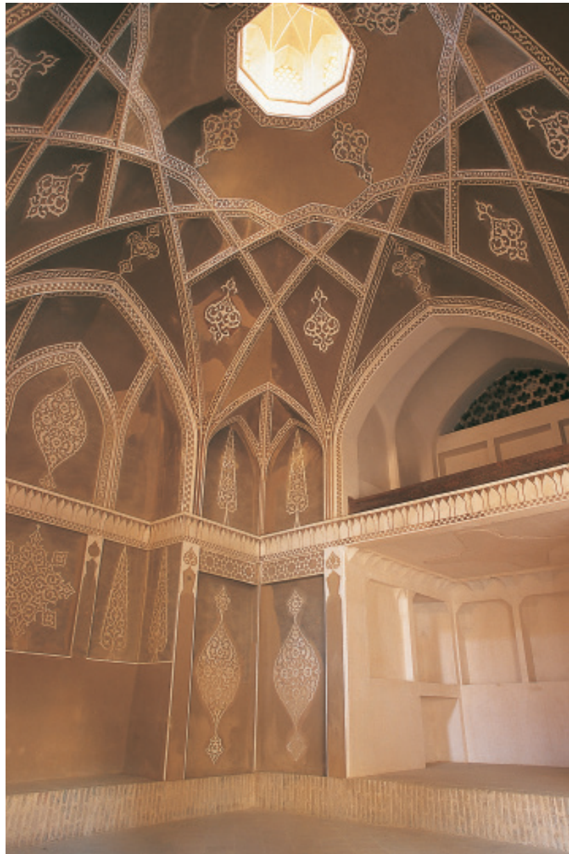
Figure 17. Covered space at the eastern corner of the first floor of the northern courtyard.
