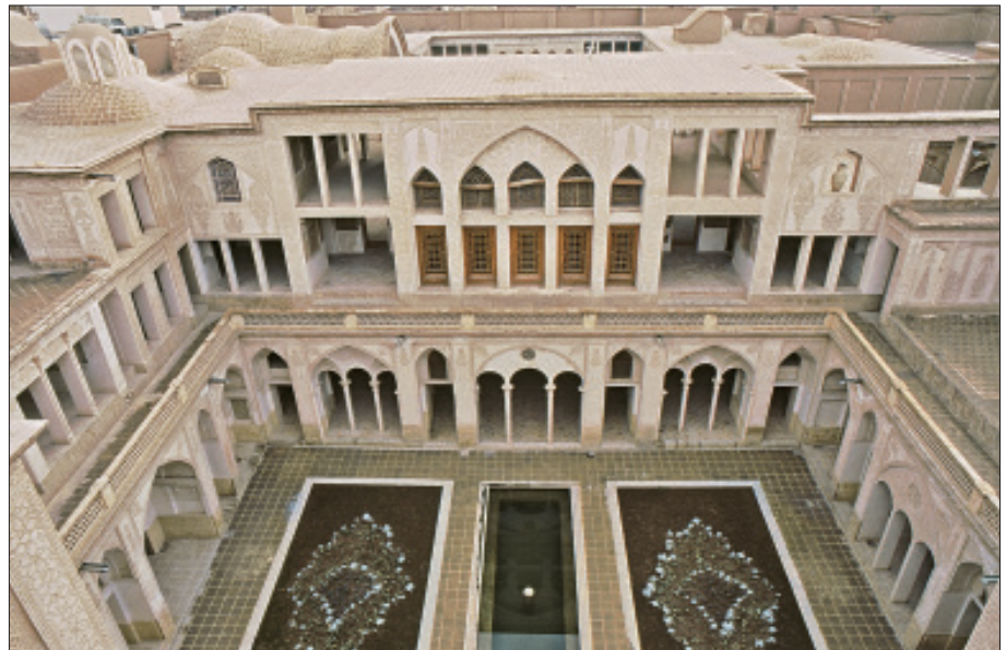
Figure 10. Southeastern side of the northern courtyard.
