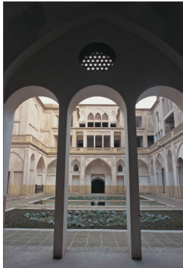
Figure 5. Northeastern façade in the northern courtyard.
