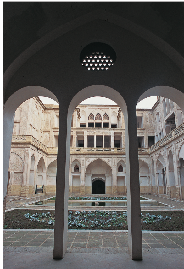
Figure 5. Northeastern façade in the northern courtyard.
