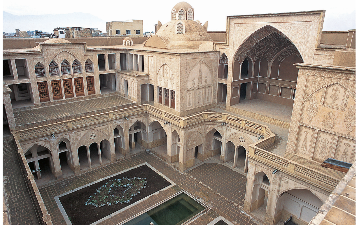
Figure 4. Northwestern and southwestern sides of northern courtyard.
