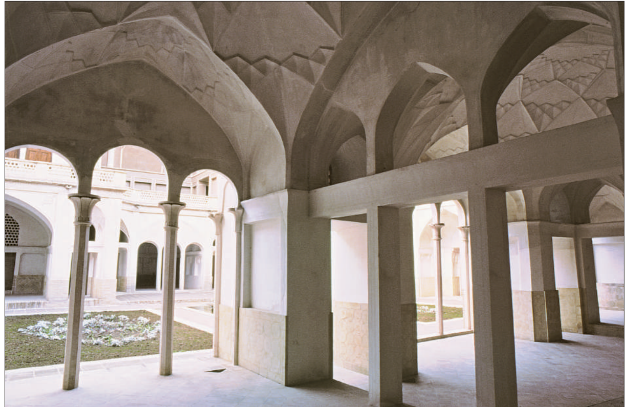
Figure 14. Western part of the space between the central and northern courtyards at the sunken garden floor level; looking toward the northern courtyard.
