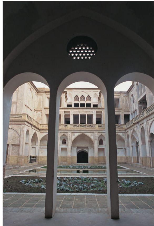
Figure 5. Northeastern façade in the northern courtyard.
