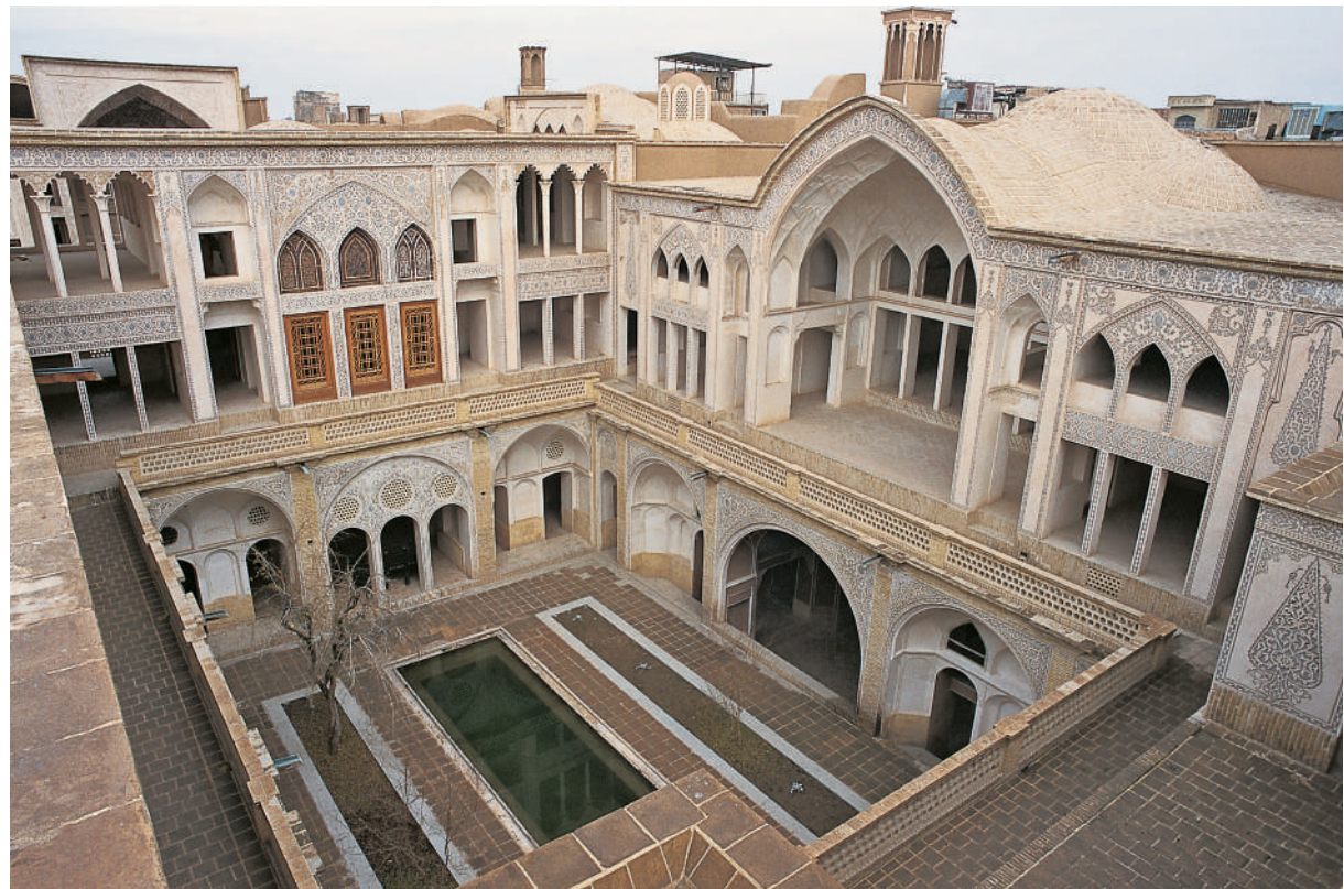
Figure 1. Northeastern and northwestern sides of the central courtyard.
